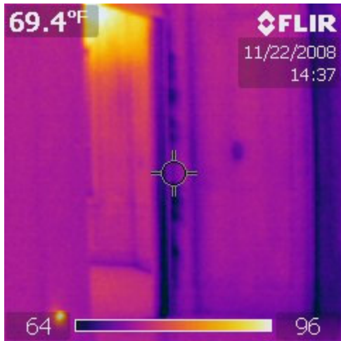
Air infiltration at the office pocket doors
